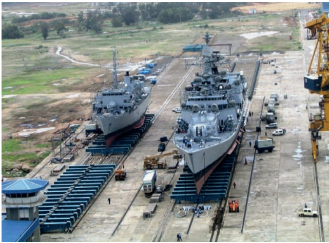
Shiplift Facility at Karwar
