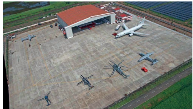
Naval Air Enclave (NAE) at the Cochin International Airport (CIAL), Nedumbassery
