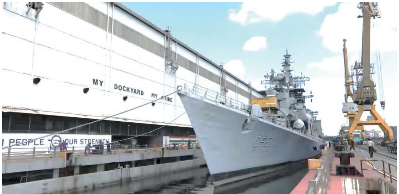
A Warship Under Maintenance at Naval Dockyard, Visakhapatnam
