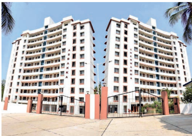
Phase II of the Married Accommodation Project at Karwar Naval Base
