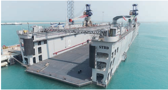
FDN-2 built by L&T
